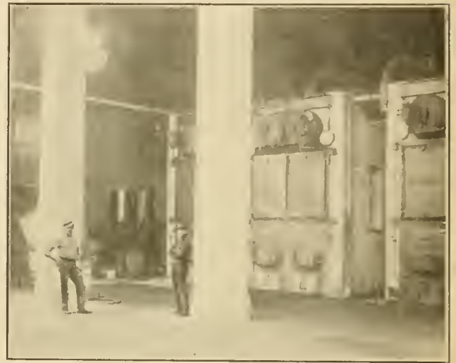
VIEW IN THE BOILER ROOM, SHOWING CONCRETE PIER CONSTRUCTION.—BABCOCK & WILCOX BOILERS.
